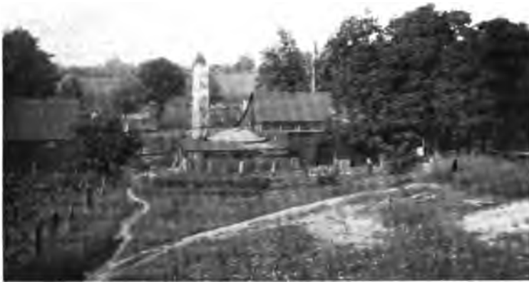
(A) Pipe works at Pamplin.
